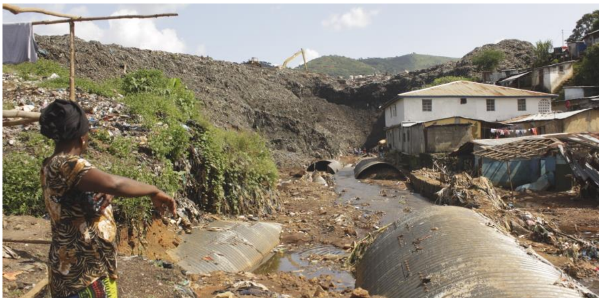
Figure 7: Bomeh dumpsite (viewed from Kissy community) is forming a dam across the river, forming a dam in the rainy season, flooding a settlement upstream; at the same time river water seeping through the dumpsite, washing out toxic materials and solid waste, contaminating downstream Kissy community (Photo: MSB/UNDP)
